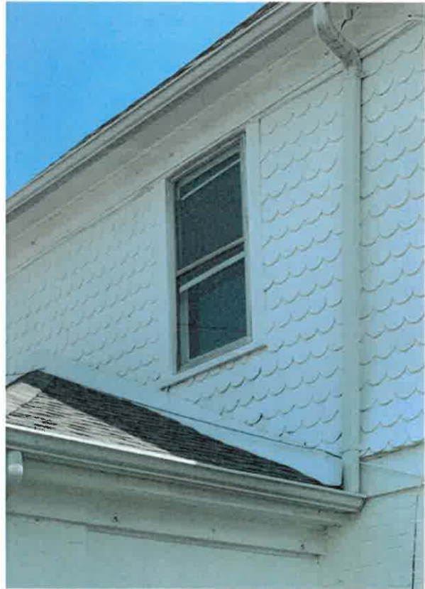
Vulnerable flashing
